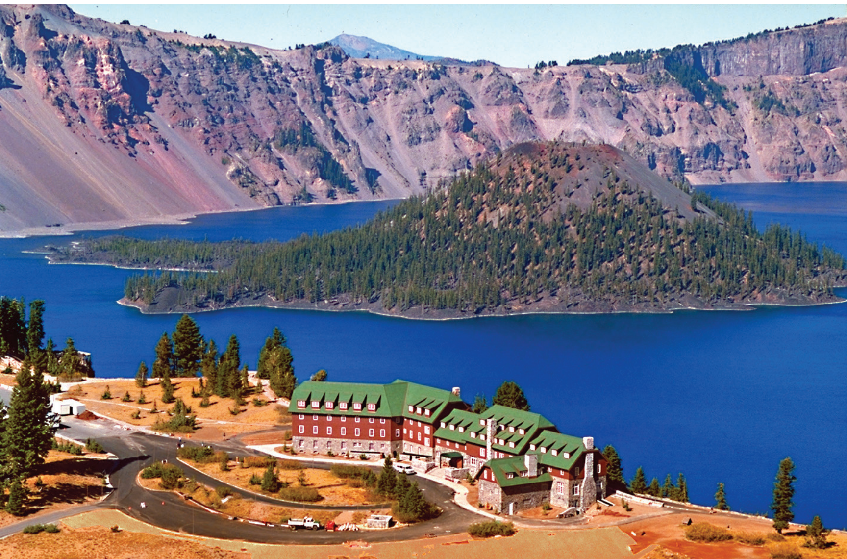
Crater Lake Lodge, Crater Lake National Park, Oregon, opened in 1915, and had extensive renovations in 1995. The work restored its historic character and preserved the classic architecture design for future generations. Photo: Courtesy of FFA Architecture and Interiors, Inc.
