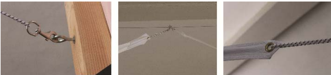
Figure 2: Photographs of installation details: eyebolt connection, sliding cable connection and fabric panel corner.
